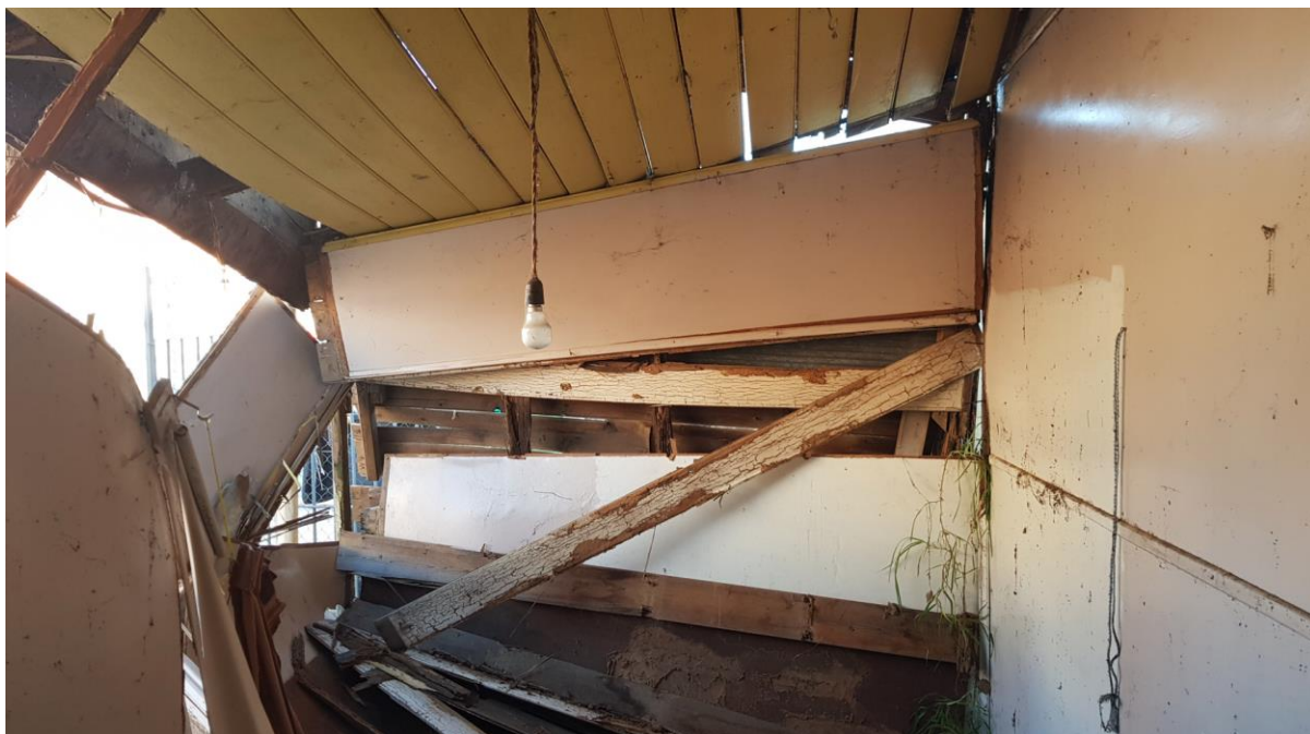
Photo 5: Rear Southern skillion has collapsed. Extensive termite damage visible.
