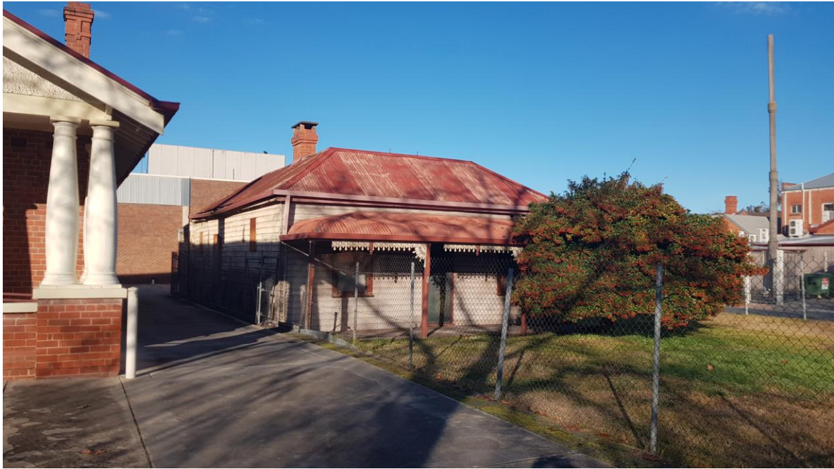
Photo 1: View from North-East. Eastern wall is directly on the boundary. Stability of masonry chimney close to Eastern neighbouring property constitutes a major safety issue.
