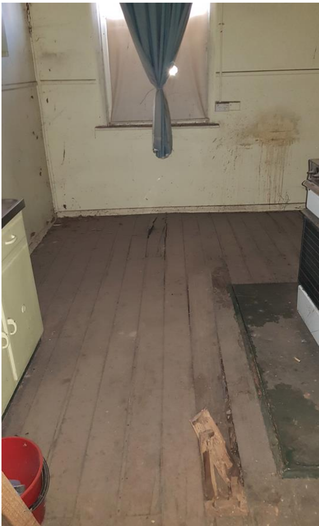
Photo 7: Floor framing is directly against the ground. Extensive floor movement and collapse exists.
