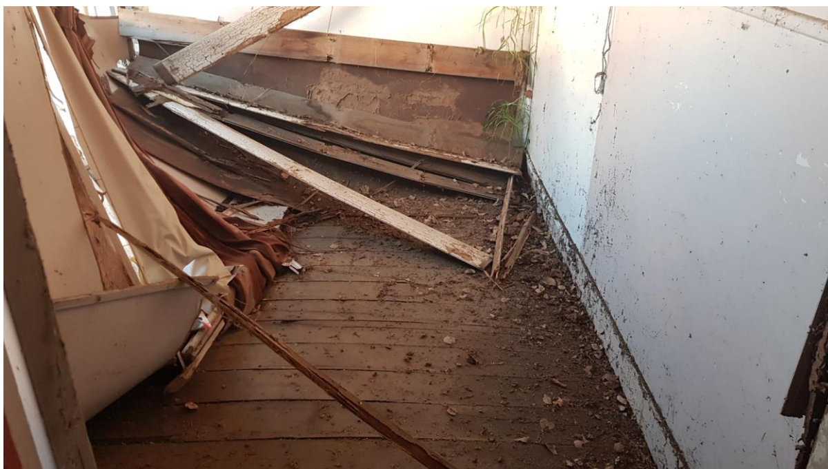
Photo 6: Rear Southern skillion has collapsed. Extensive termite damage visible.
