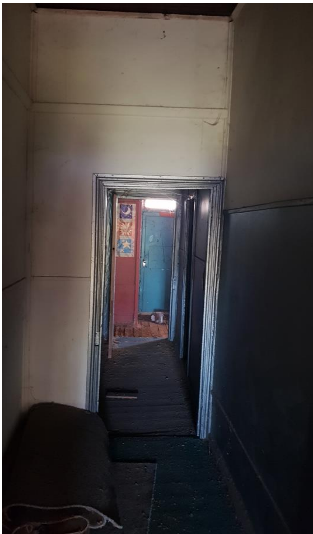
Photo 8: Extensive movement to floors, wall framing, doors, and windows throughout.
