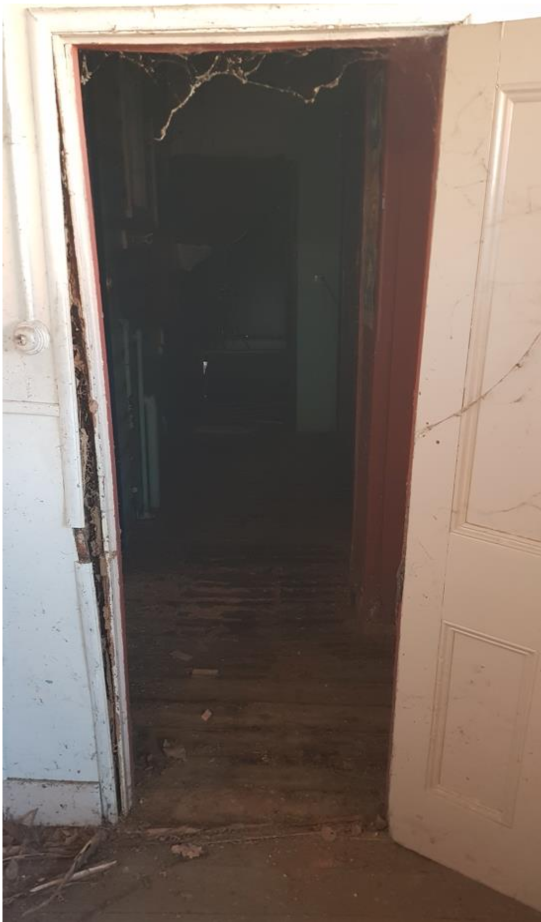
Photo 9: Extensive termite damage throughout.
